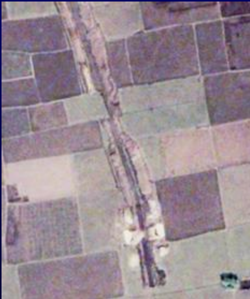
Canal under construction
