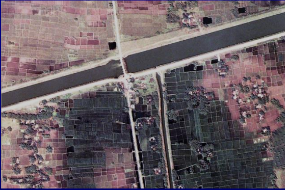
Completed section i.e., canal in place
